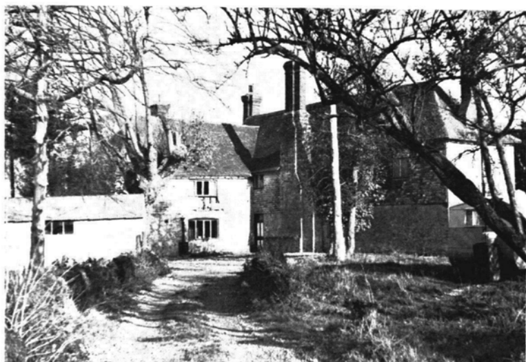
A. Harringe Court, view from the south-west.
