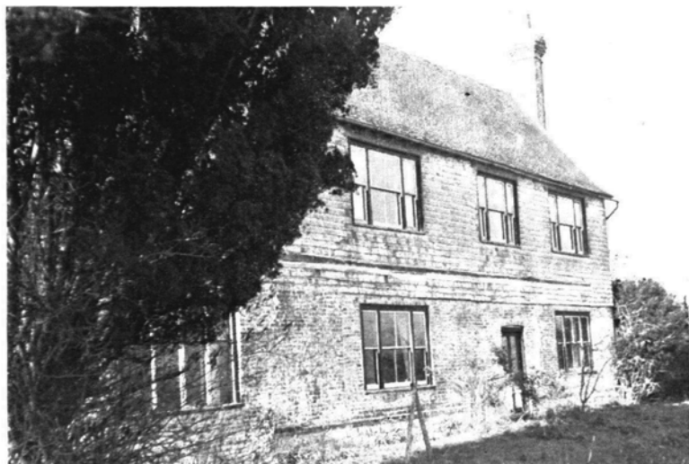
B. View of the east side.
